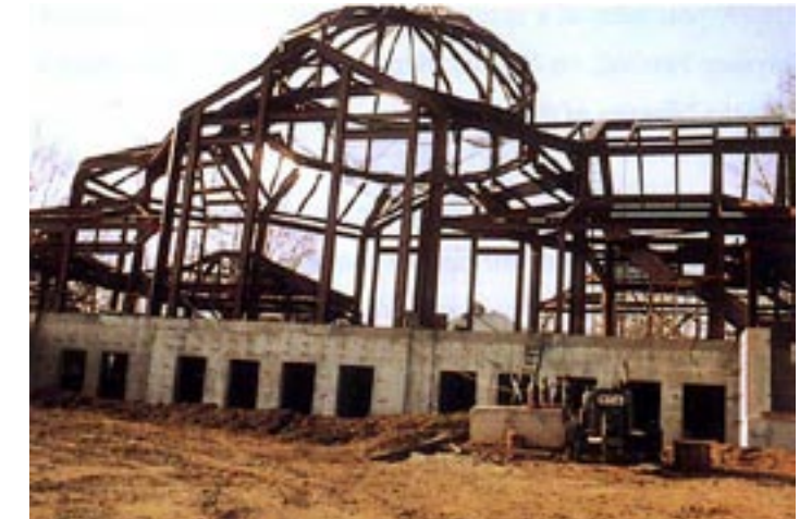
Above: Saint Barbara Greek Orthodox Church 480 Racebrook Road during construction
